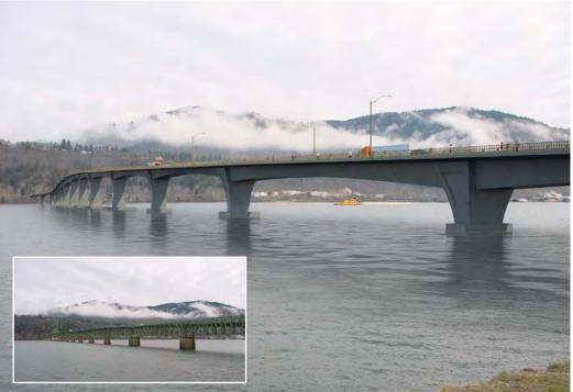
The segmental box girder option is a single box girder of varying depth constructed of concrete. This includes two 12-foot travel lanes and 8-foot shoulders, providing for a wider and safer crossing. This option has a main span of 500 feet that will yield 450 feet of horizontal navigation clearance. Segmental box girder approach spans with lengths varying from 100 feet to 400 feet will comprise the remainder of the bridge.
