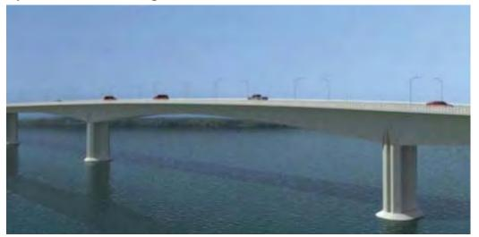
Example rendering of a concrete segmental box girder bridge.
