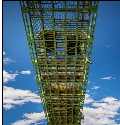
The current bridge decking is steel grate.
