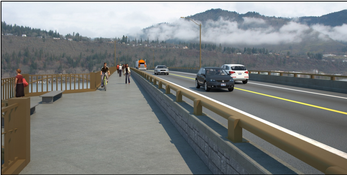
The proposed bridge will have 12-ft. wide travel lanes, 8-ft. wide shoulders, and 12-ft. dedicated bike/pedestrian facility.
