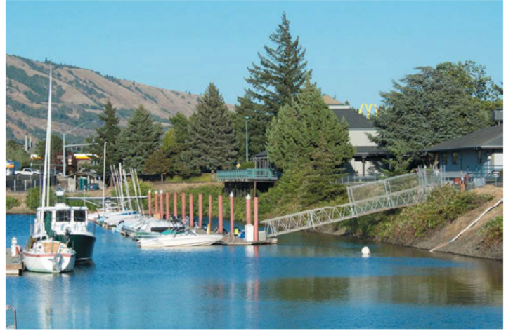
The South Basin Dock will be upgraded and expanded in 2024-25
