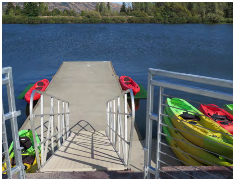
Existing Conditions at Site
