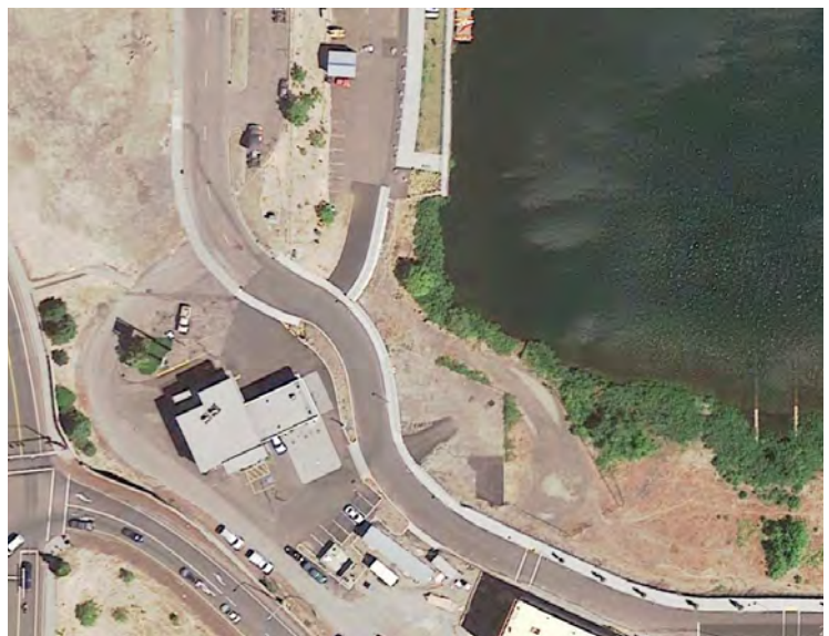
Existing Conditions at Site
