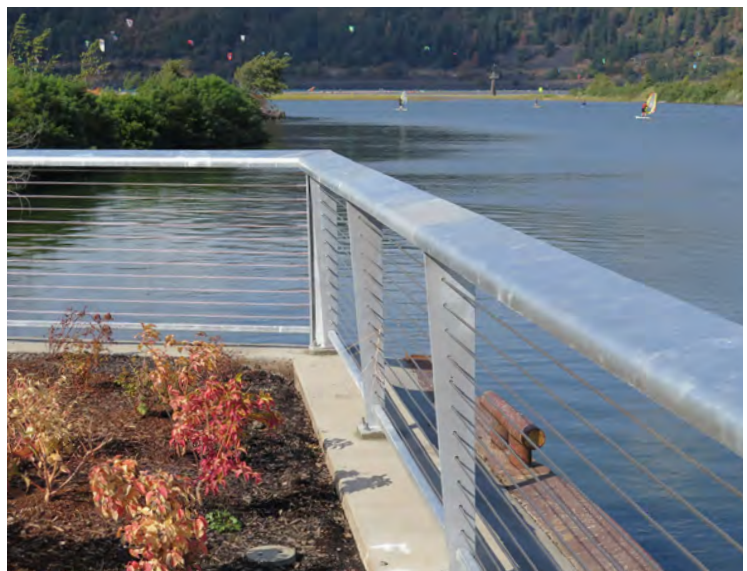
Existing Conditions at Site
