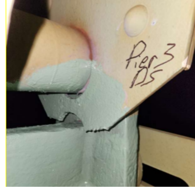
ROCKER BEARING MODIFICATIONS- REPAIR #6
