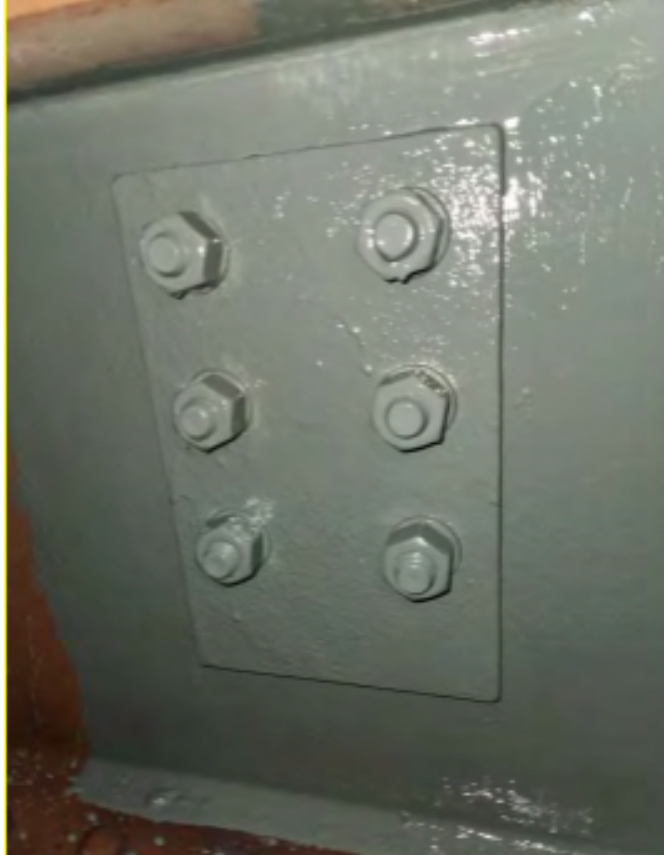
FLOORBEAM KNEE BRACE REPAIR- REPAIR #4
