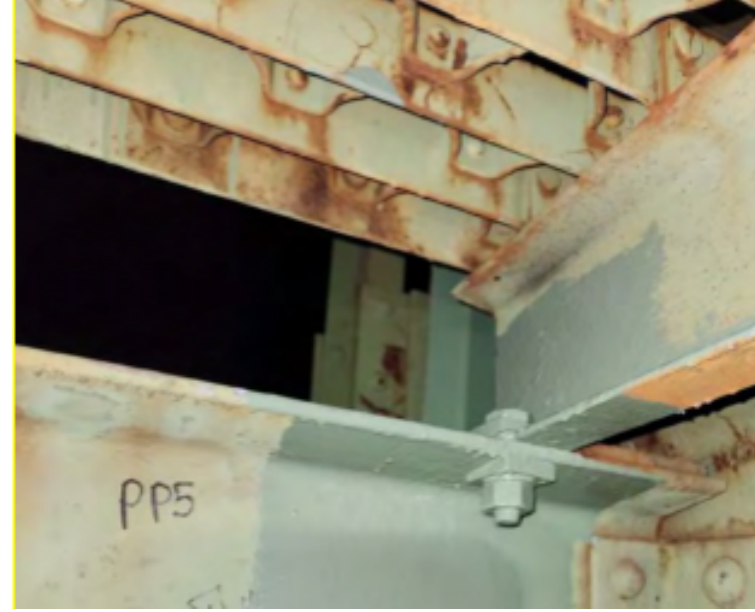
STRINGER TO SUB-STRINGER REPAIR #2
