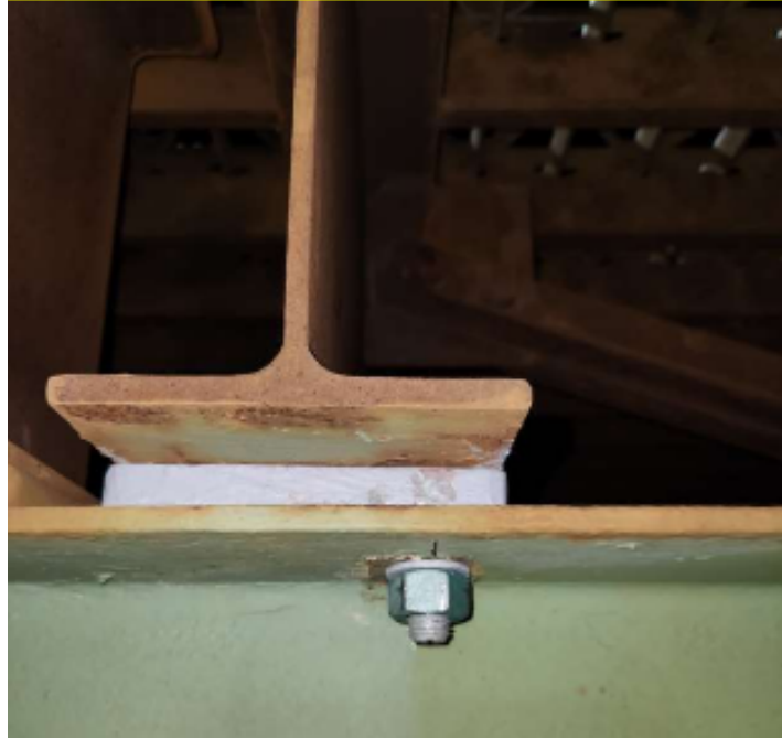
STRINGER TO FLOOR BEAM CONNECTION REPAIRS
