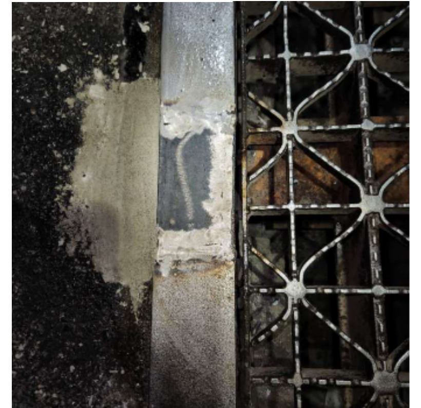
JOINT HEADER REPAIR
