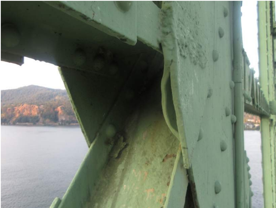
IM06645_D5: Welded Gusset Plate at M7 of Span 11 US
