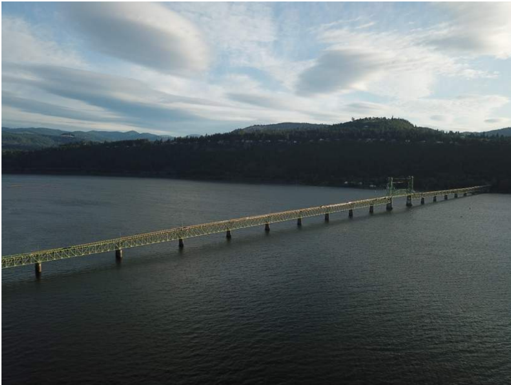
IM06645_A1: Elevation Looking Northwest (photo courtesy of 2020 inspection)
