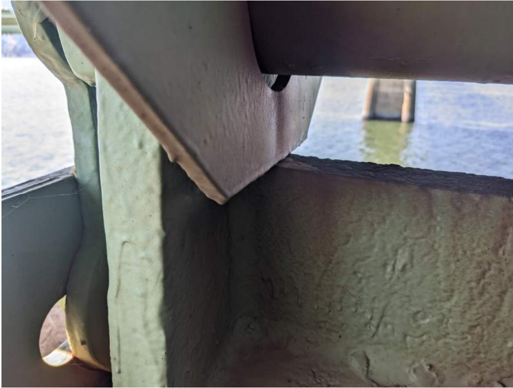
IM06645_E6: Vertical Gusset Bearing on Rocker Stiffener at Span 15 Pier 16 DS
