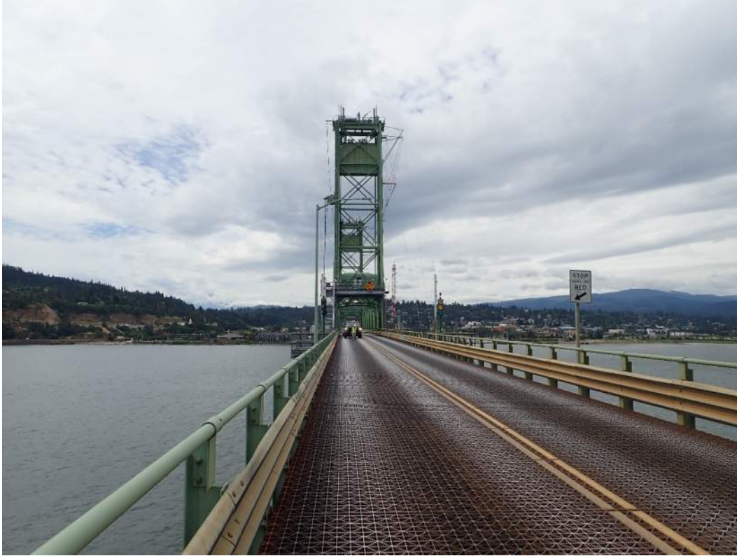
IM06645_A0: Roadway Looking South (photo courtesy of 2020 inspection)
