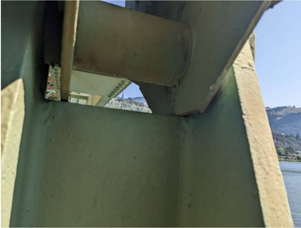
IM06645_E8: Vertical Gusset Bearing on Anchor Stiffener at Span 16 Pier 16 US
