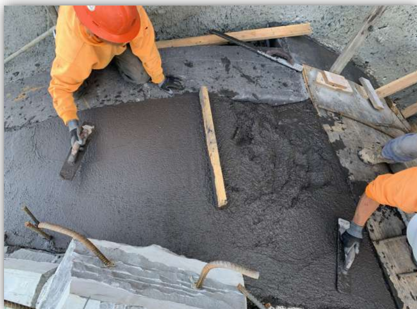
Concrete Forming and Pouring at West Portal of Tunnel
