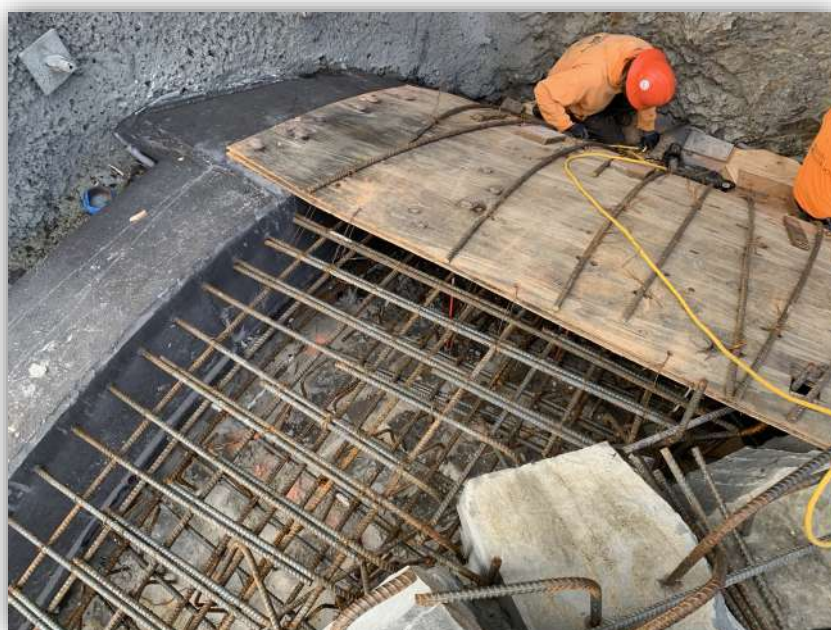
Concrete Forming and Pouring at West Portal of Tunnel
