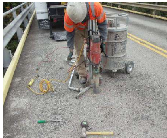
Figure 2. Core Drilling Apparatus
