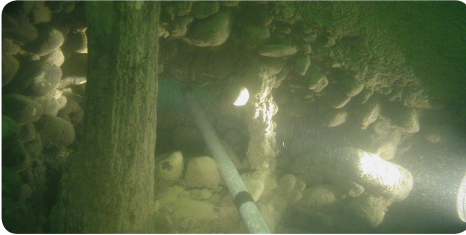
Pictured above and to right: Underwater inspections of bridge piers show deterioration, evident in concrete voids, anchorage system corrosion, scour at the mudline and scaling at the waterline.
