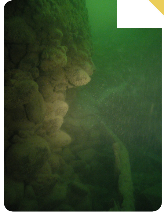
Pictured above and to right: Underwater inspections of bridge piers show deterioration, evident in concrete voids, anchorage system corrosion, scour at the mudline and scaling at the waterline.
