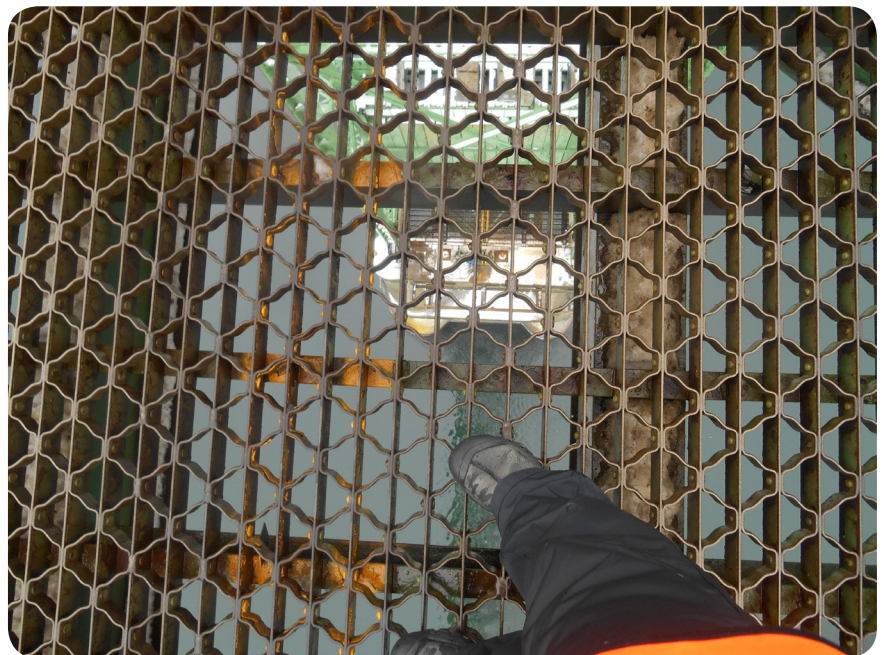
Pictured above: The bridge's nearly mile-long grated steel deck presents an environmental hazard to the Columbia River, as there is no barrier to trash, debris, and fluids from motor vehicle traffic. The deck requires bi-annual maintenance welding, which causes significant traffic delays.
