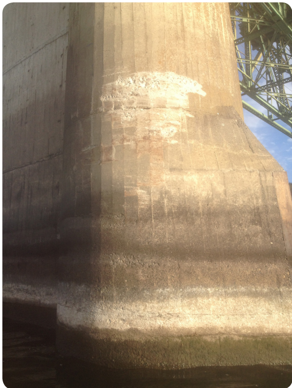
Pictured above: Evidence of a large single, or multiple allisons is seen on the north lift span pier. This bridge is well known as the most often struck object in the entire Columbia-Snake River system.
