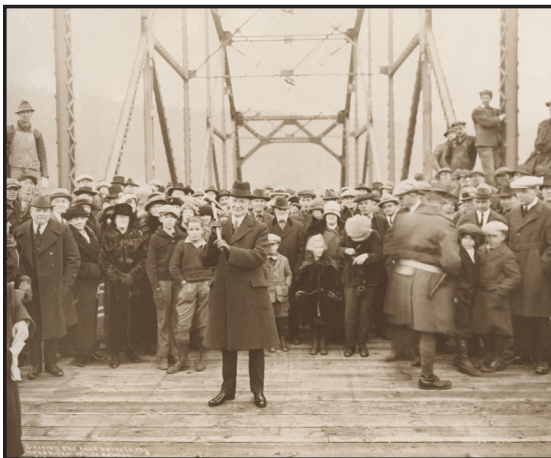
Leslie Butler driving the last spike in the wooden bridge deck December 6, 1924.
