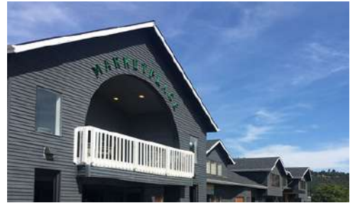
Marketplace office and hotel suites at the Hood River Inn east of the existing bridge in Oregon.
