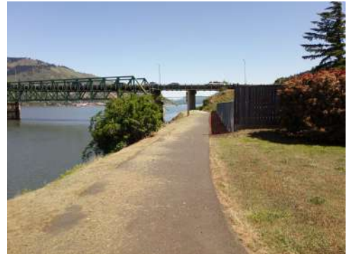
Waterfront Trail crosses under the existing Hood River Bridge.
