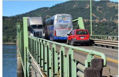
Narrow lanes and the steel grated bridge deck create uncomfortable driving conditions.
