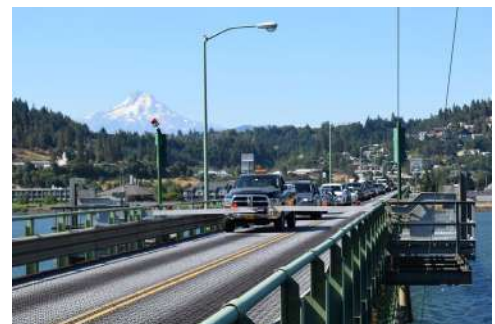
The existing lift span results in traffic delays.
