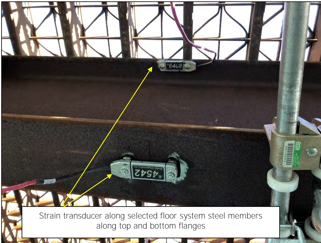
Figure 2 – Strain transducers along selected Span 2 floor system members (typical)
