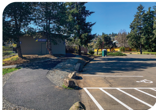
New ADA ramp at the Marina restrooms.
