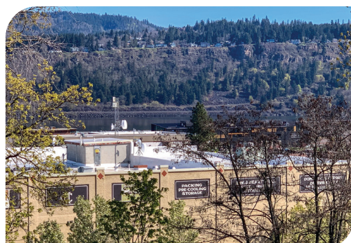
Big 7 building’s re-roof.
