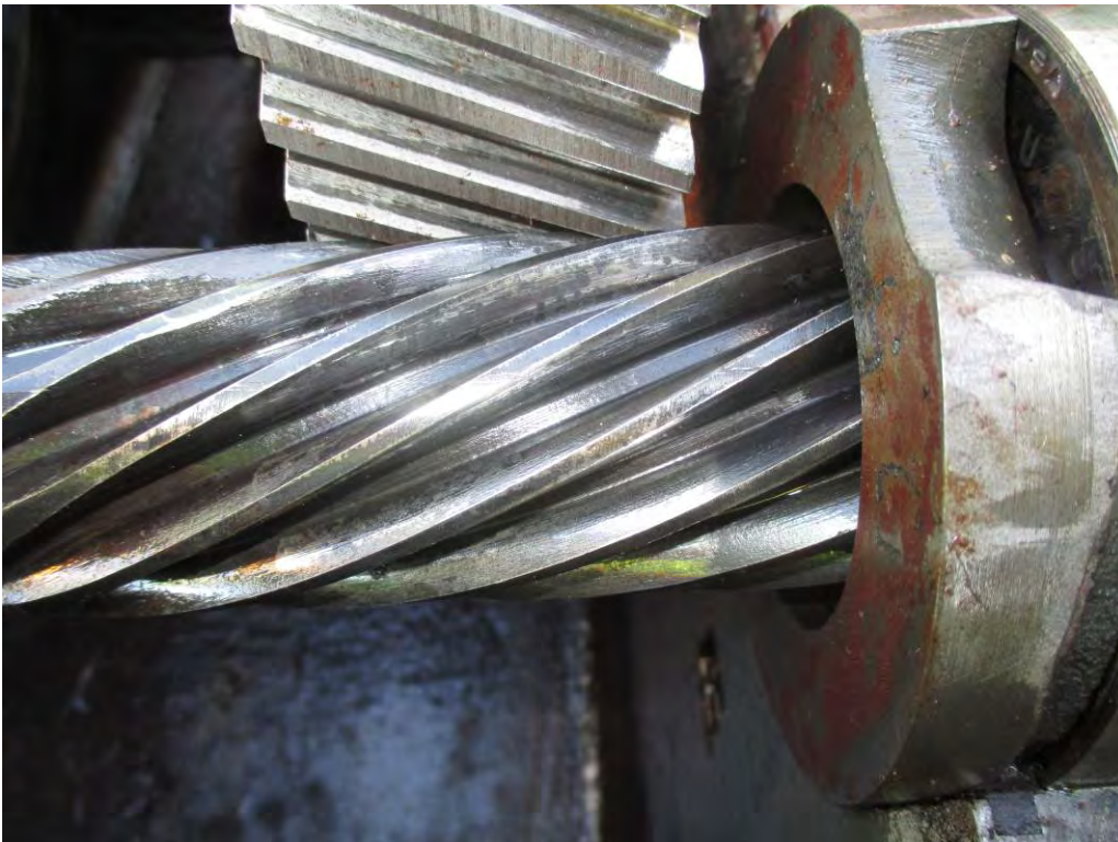
Photo 14. South Primary Reducer. View of east first reduction gear set, opening face of pinion teeth. Note the pits on the outboard (right) end of the teeth.
