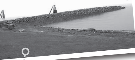
Jetty and beach repairs completed at Event Site
