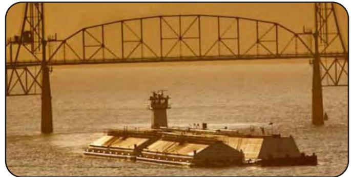
Navigational clearance on the federal waterway is at least 200' less than the minimum recommended width.
