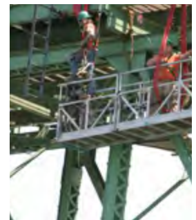
The bridge exits in a very hostile marine environment requiring near constant maintenance.
