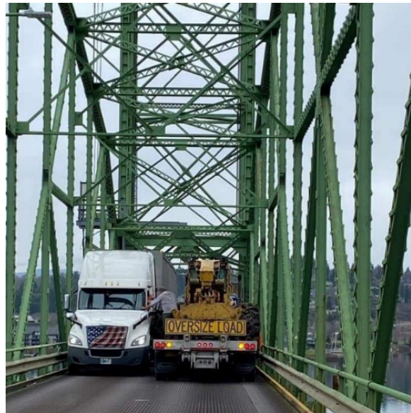
Figure 2-6: Narrow Lanes and Trucks Conflict
