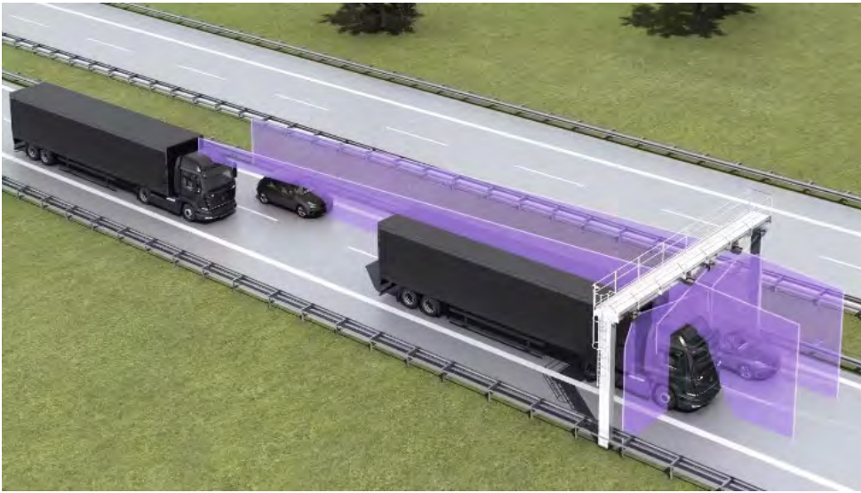
Figure 4: LiDAR based vehicle detection system for over height and over width vehicles (SICK Free Flow Profiler, 2024)
