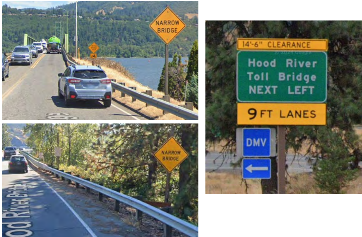
Figure 5: Existing warning signs for horizontal clearance (Google Maps, 2024)
