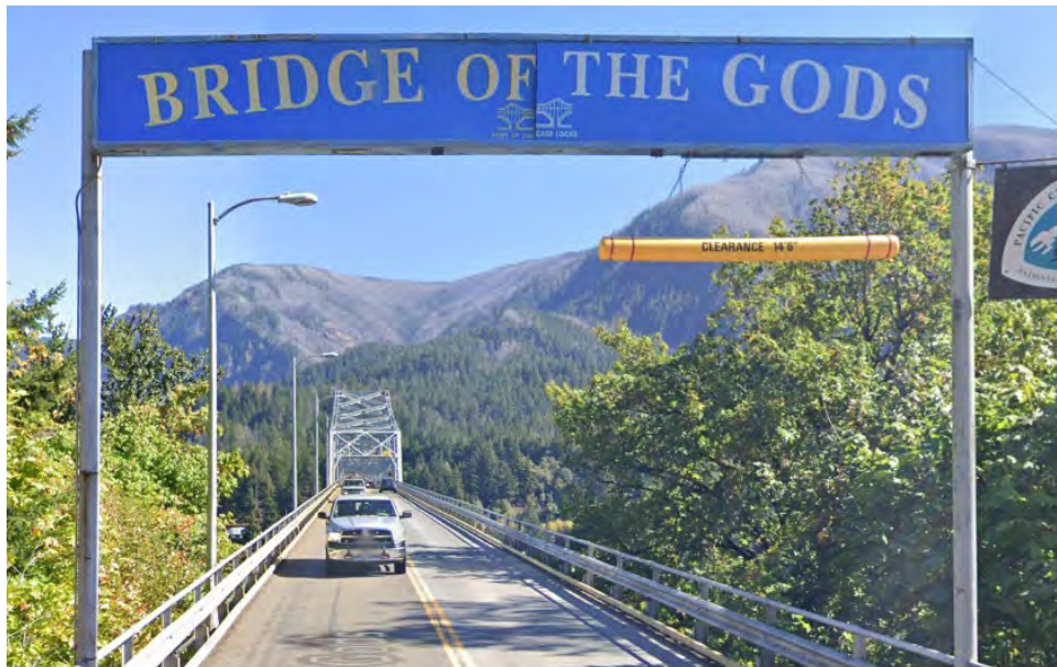
Figure 2: Flexible vertical clearance bar at Bridge of the Gods, Washington Approach (Google Maps, 2021)
