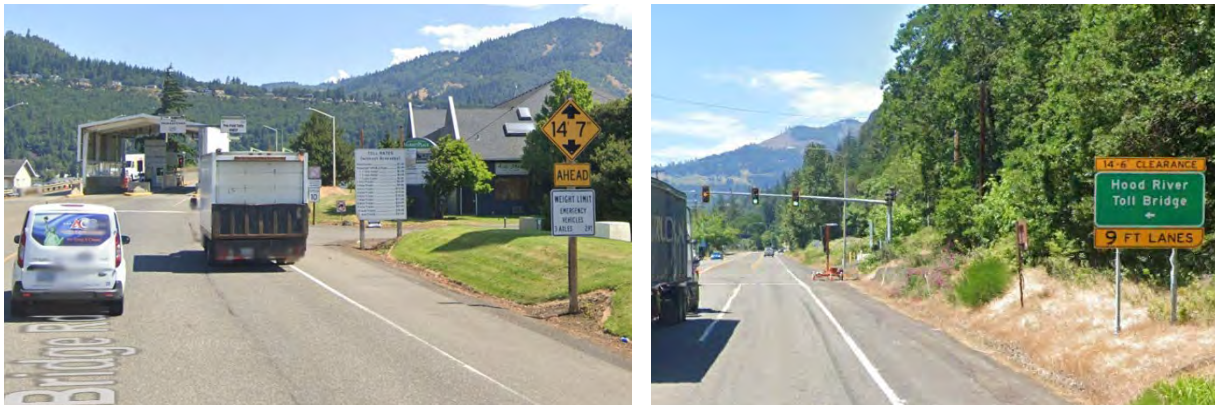
Figure 1: Existing advance clearance warning signs in Oregon side (Left) and Washington Side (Right) (Google Maps)
