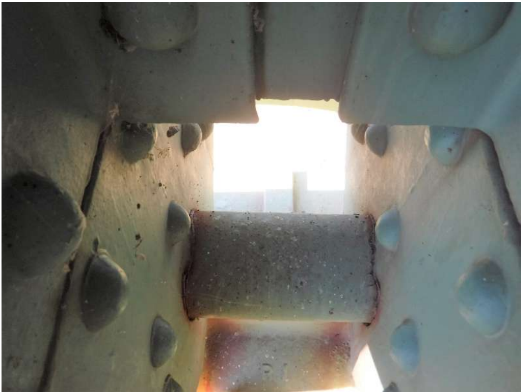
Photo 2 – Typical Mushrooming of Flange at Pin
