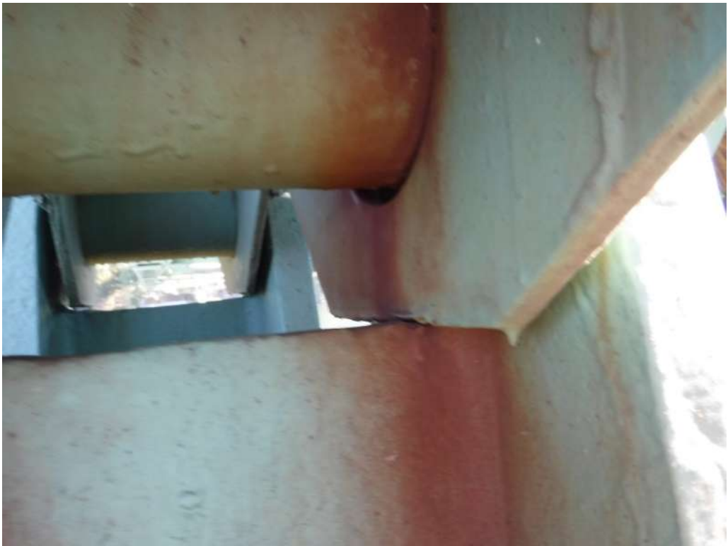
Photo 6 – Bearing on Rocker Close-up
