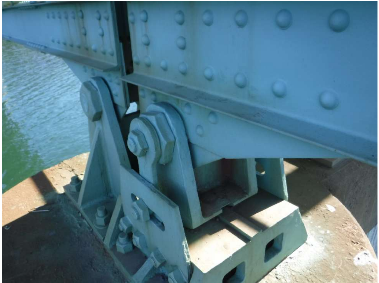
Photo 1 – Typical Rocker Bearing
