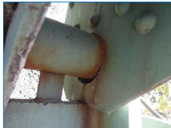
Figure 2. Rocker bearing at Pier 20
