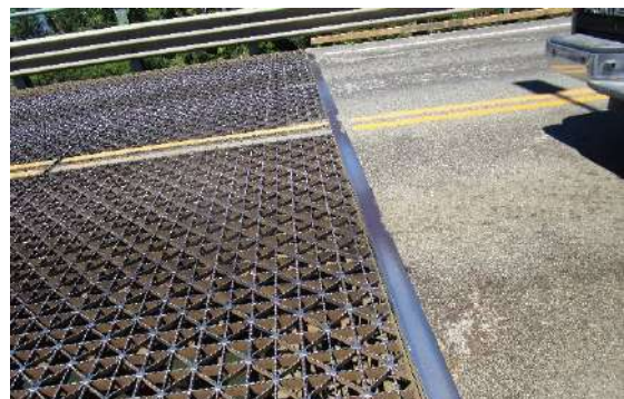
Figure 1. Joint at Pier 20
