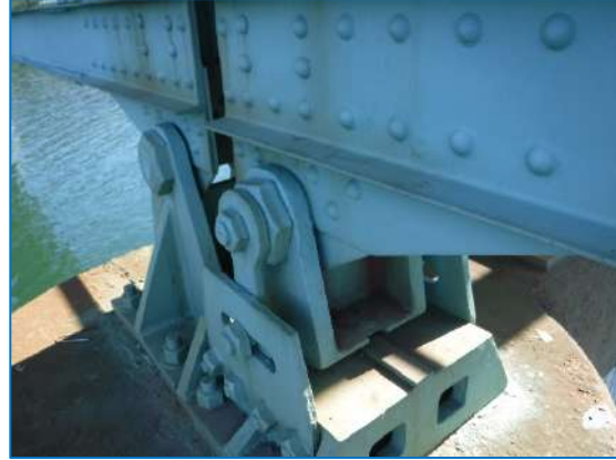
Figure 4. Typical fixed and expansion bearings
