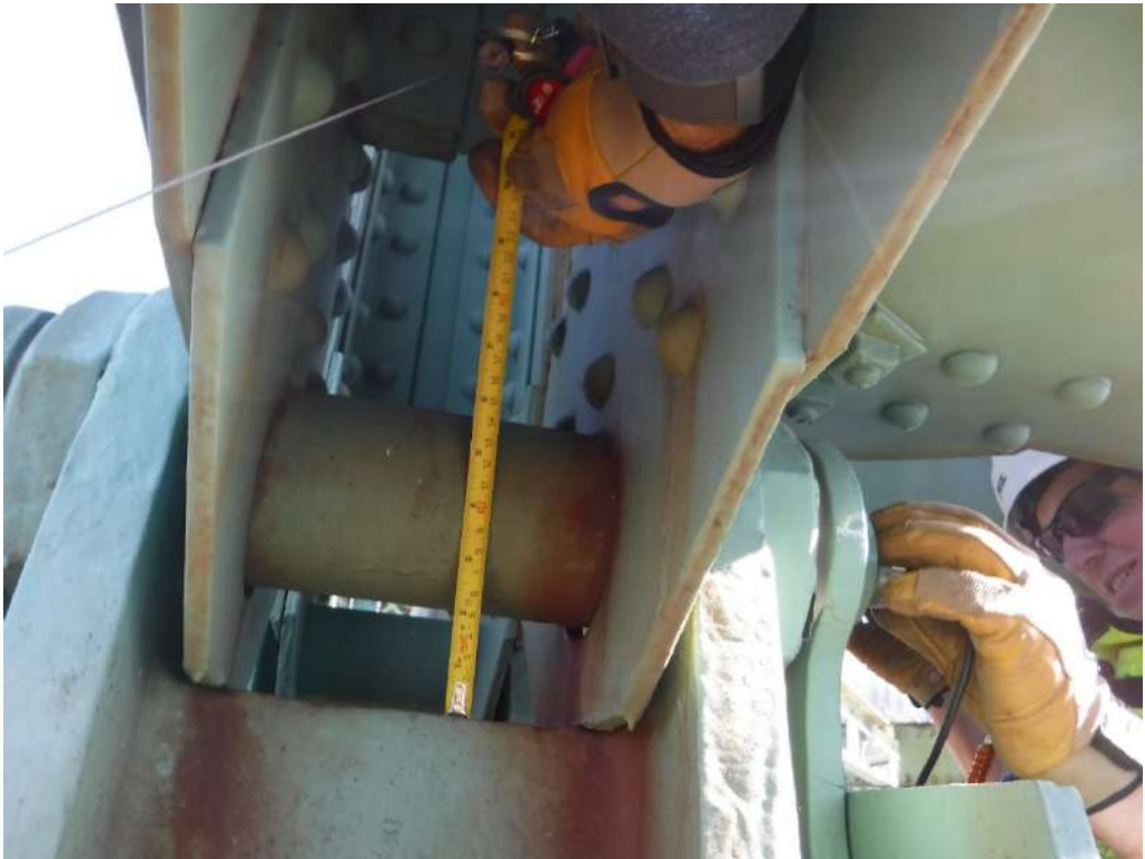
Photo 5 – Bearing on Rocker – Typical
