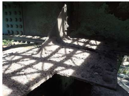
Figure 9. Debris accumulation
