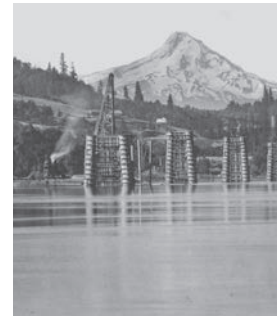
The Hood River-White Salmon Interstate Bridge under construction in 1923
