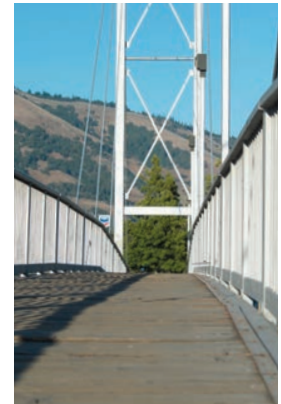
Pedestrian Bridge over the Hood River will receive a new deck and new lighting in 2022
