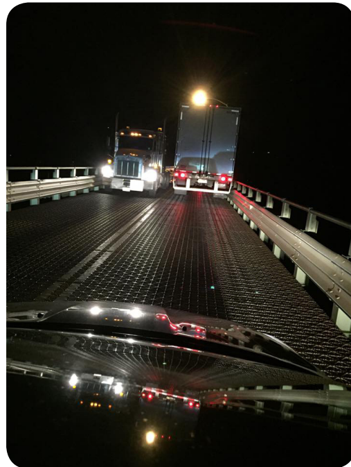
The truck on the right scrapes the guardrail while negotiating a crossing with another truck approaching.
