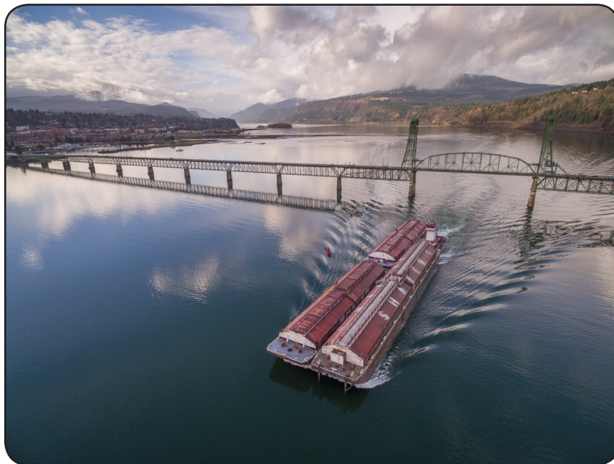
In this view looking downstream of the Columbia River federal waterway, a typical barge tow navigates the narrow span of the Hood River Interstate Bridge.
