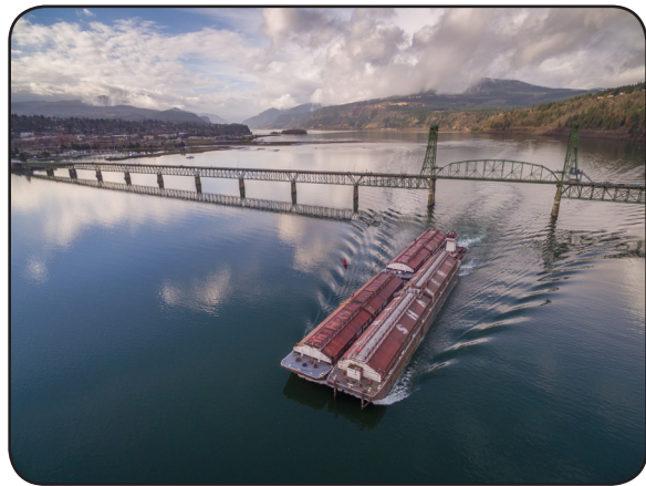
The current lift span is more than 200’ narrower than the minimum recommendation.
