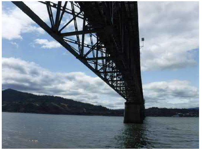
Photo 4. Existing bridge facing south from WA side
