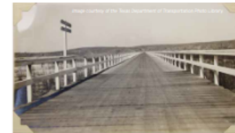
The Charlie Walters Bridge, a wooden trestle bridge constructed in the 1920s.
