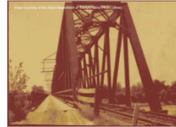
Kansas, Oklahoma & Gulf Railroad bridge over the Red River at Carpenters Bluff, early 1900s.
