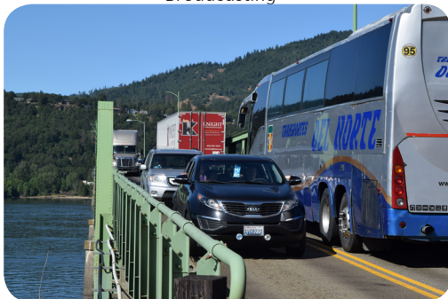
Large trucks, busses, and passenger vehicles crossing within inches of each other.
