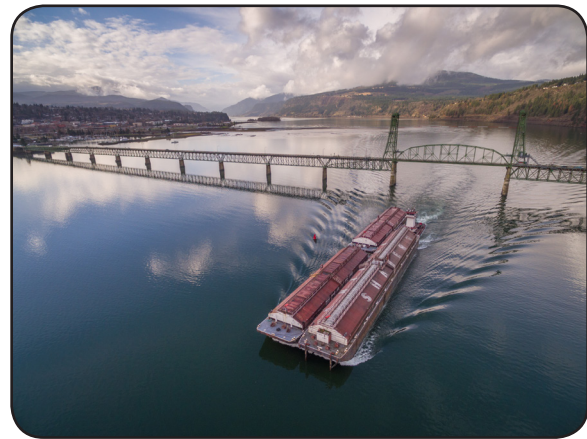
The current lift span is more than 200’ narrower than the minimum recommendation.
