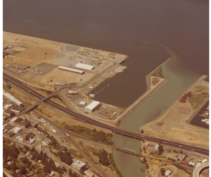
The third fill project, in the Marina Park area (right), was completed in 1970 and the area's general improvements began.
