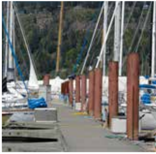
The Hood River Marina underwent an electrical upgrade in 2013
