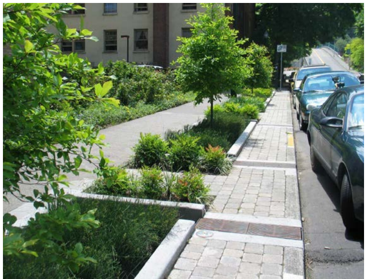
Stormwater Treatment Example
