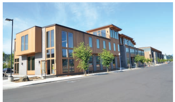
Business development since 2010 has dramatically changed Portway Avenue.
