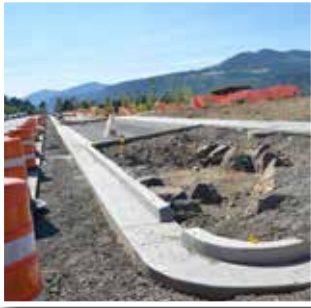
Parking improvements underway during the summer of 2013
