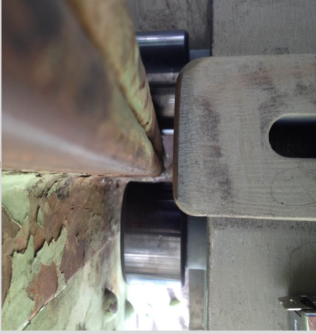
2016 Span Guide Replacement & Repairs
