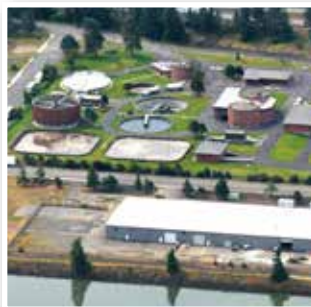
Hood River sewage treatment plant
