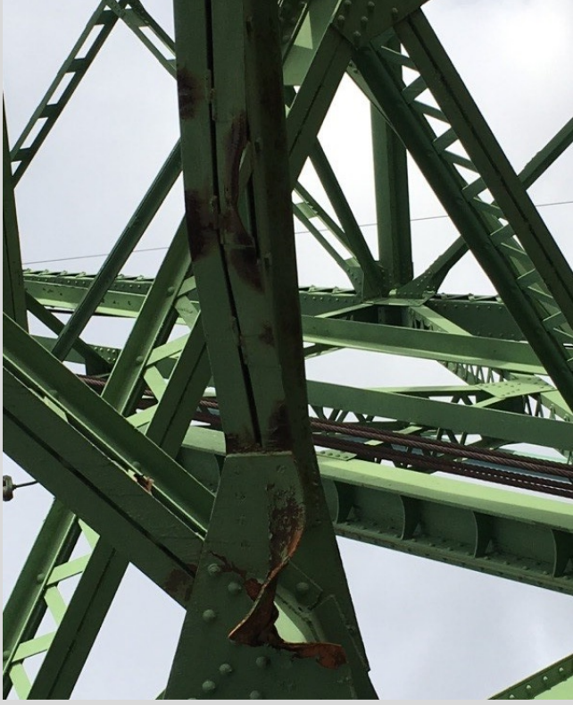
2019 Portal Truss Repair
