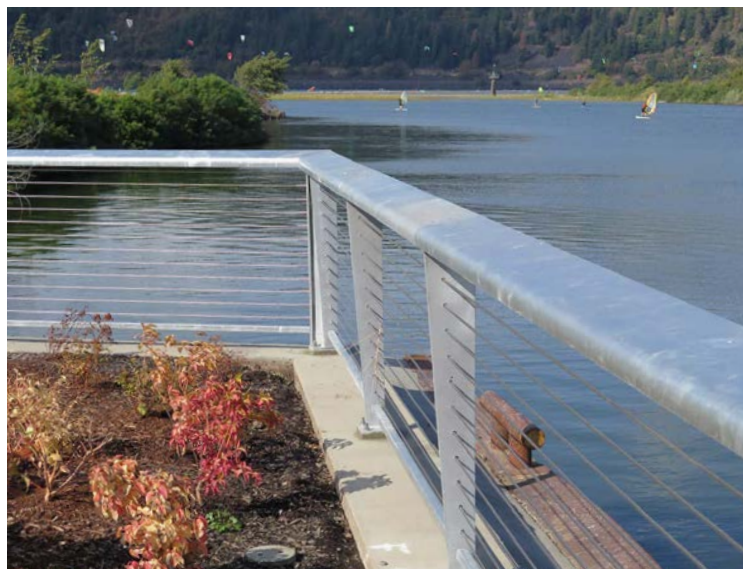
Existing Conditions at Site
