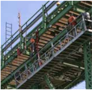
Hood River Bridge maintenance
