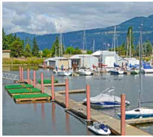
South Dock at the Marina
