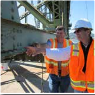
The 90 year old Hood River Interstate Bridge requires regular maintenance
