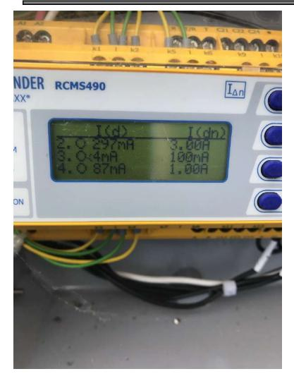
Boat houses were running ~300mA and Dock B ~90mA, with protection set to 3A and 1A respectively.
