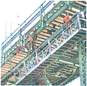
Hood River Bridge maintenance
