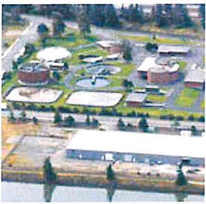
Hood River sewage treatment plant
