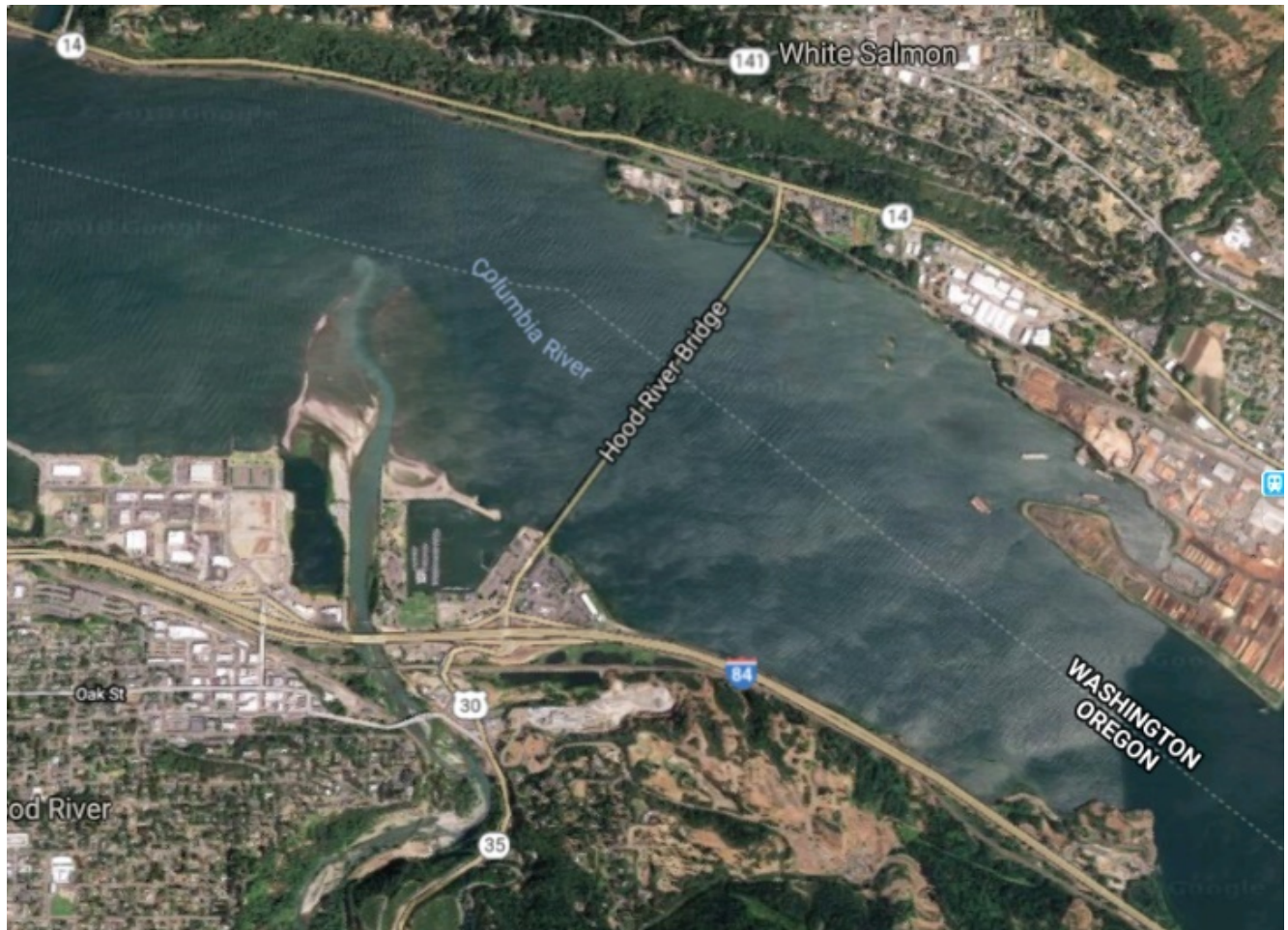
Figure 1 – Aerial Image of Hood River Bridge
