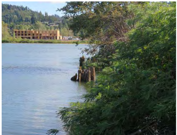
Existing Conditions at Site
