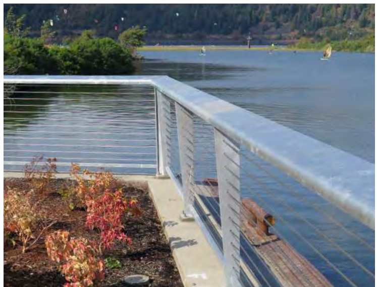
Existing Conditions at Site
