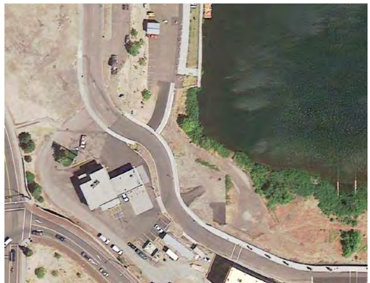
Existing Conditions at Site
