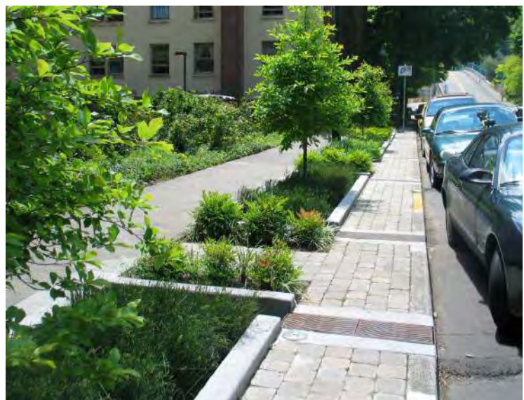
Stormwater Treatment Example
