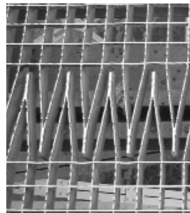
The old deck's square grid hits tires straight on, creating noise.
