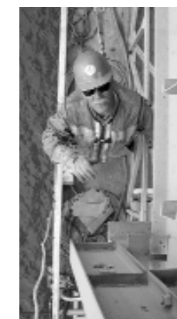
To date, most work has taken place underneath the bridge deck.
