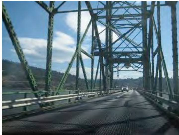
Figure 2 – The Hood River Bridge is very narrow, providing less than 10 feet in width in each travel direction.
