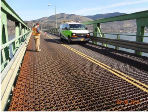
Figure 5. Oregon Spans 1-3 partial through trusses.
